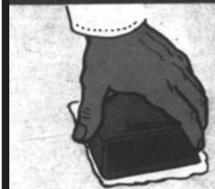
Place marker on previously determined position, applying slight pressure to force small epoxy bead around marker.
